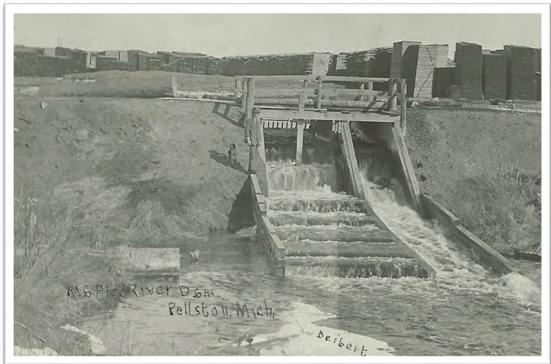
The spillway from the Pellston Mill Pond which was made by damming the west branch of the Maple River.
